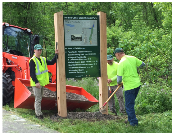
Installation of new wayfinding sign near the Limestone Aqueduct Pedestrian Bridge
