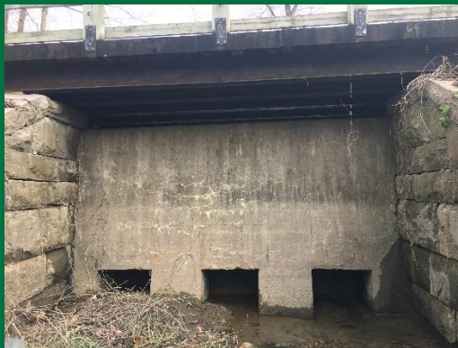
Backside of control structure
