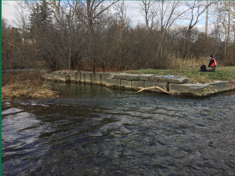
Front of Sluice Gate
