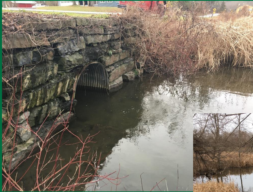
Enters via culvert
