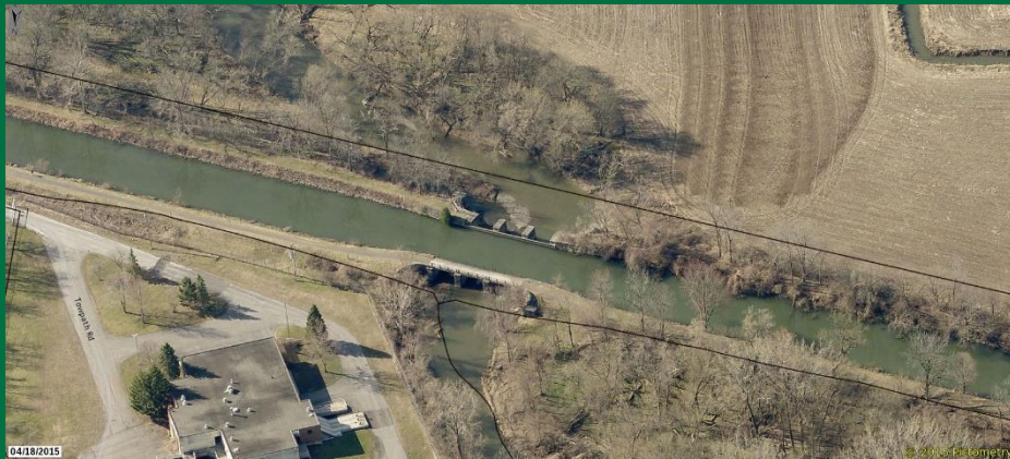
Conveys canal over Chittenango Creek
