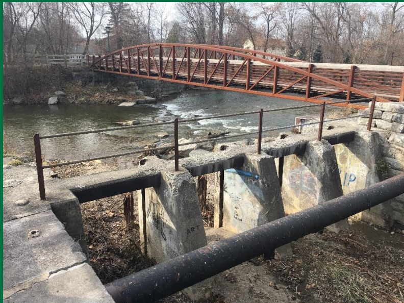
Sluice Gate with location of removed dam in background
