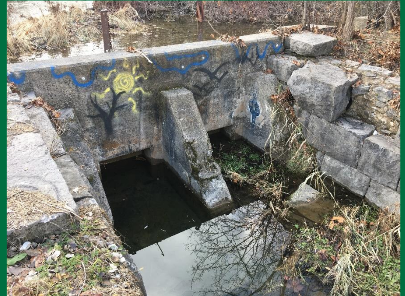
Backside of Sluice Gate
