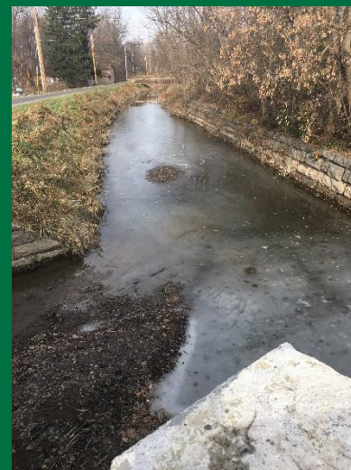
Channel conveys flow well
