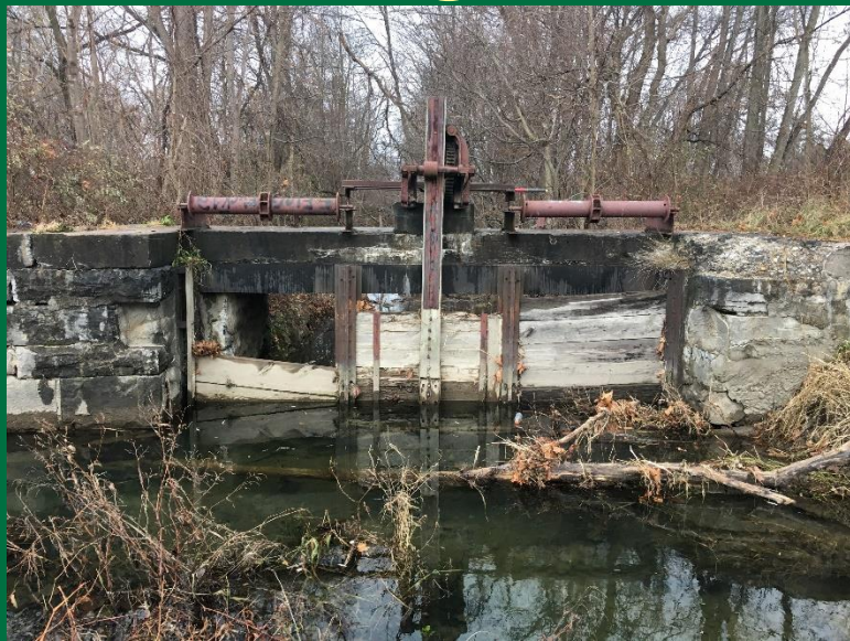
Front side of sluice gate
