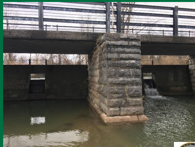
Flashboards – 1 outfall blocking outflow
