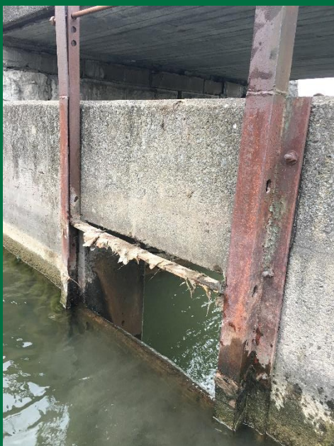
Outfall gate partially closed
